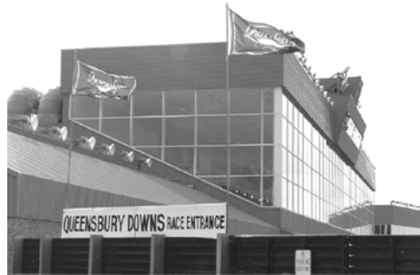
Steel Grandstand – Good Quality (A)
