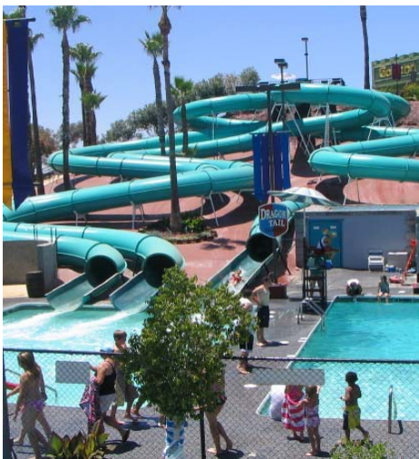
Supported Enclosed Tubular Flume
