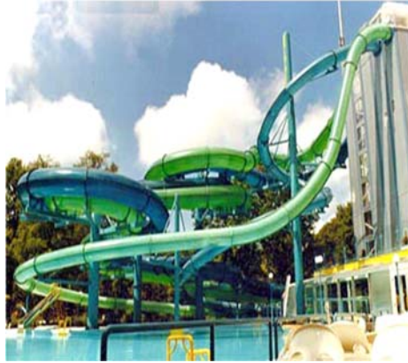
Supported Water Slide
