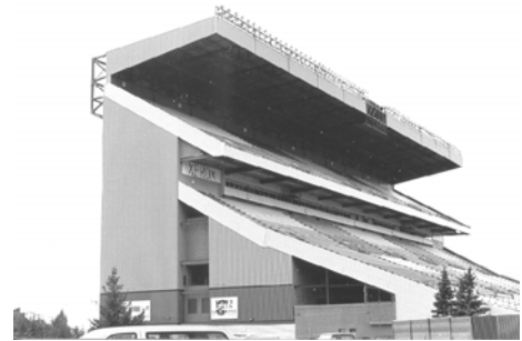
Steel Grandstand – Good Quality (A)
